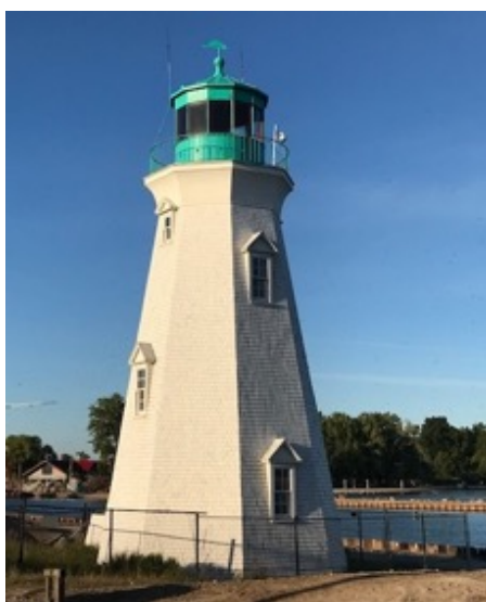
Inner Range Lighthouse 1898 with chainlink fencing
