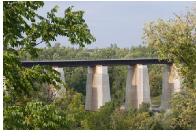
GTR Viaduct, Georgetown
